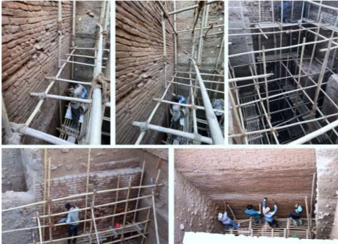
Figure 12: Simultaneous conservation of excavated structural remains
