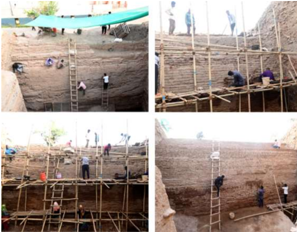
Figure 11: simultaneous conservation of excavated structural remains
