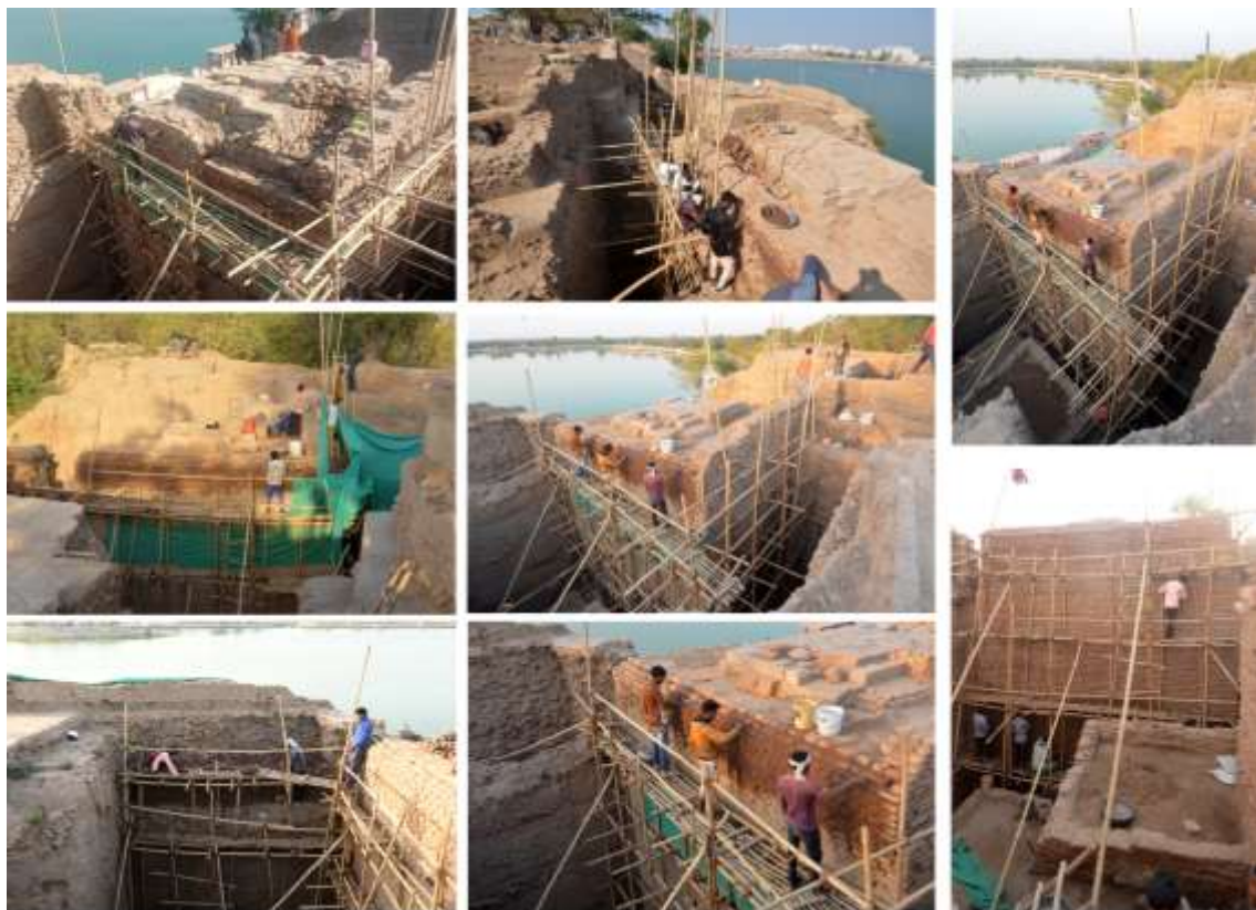
Figure 14: Consolidation of high-raised platform
