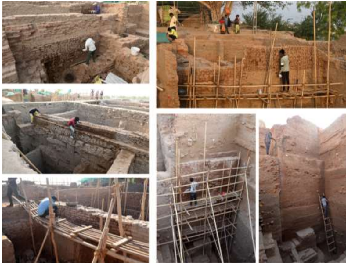
Figure 15: Consolidation of excavated structures
