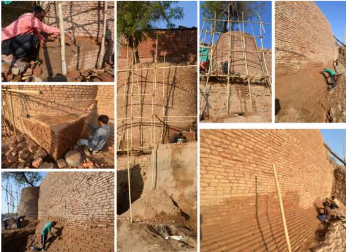
Figure 19: Consolidation of the exterior of fortification wall with traditional methods
