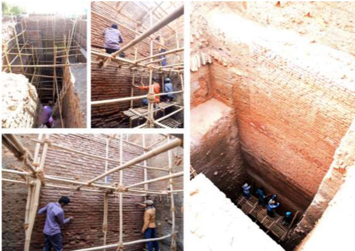
Figure 13: Simultaneous conservation of excavated structural remains
