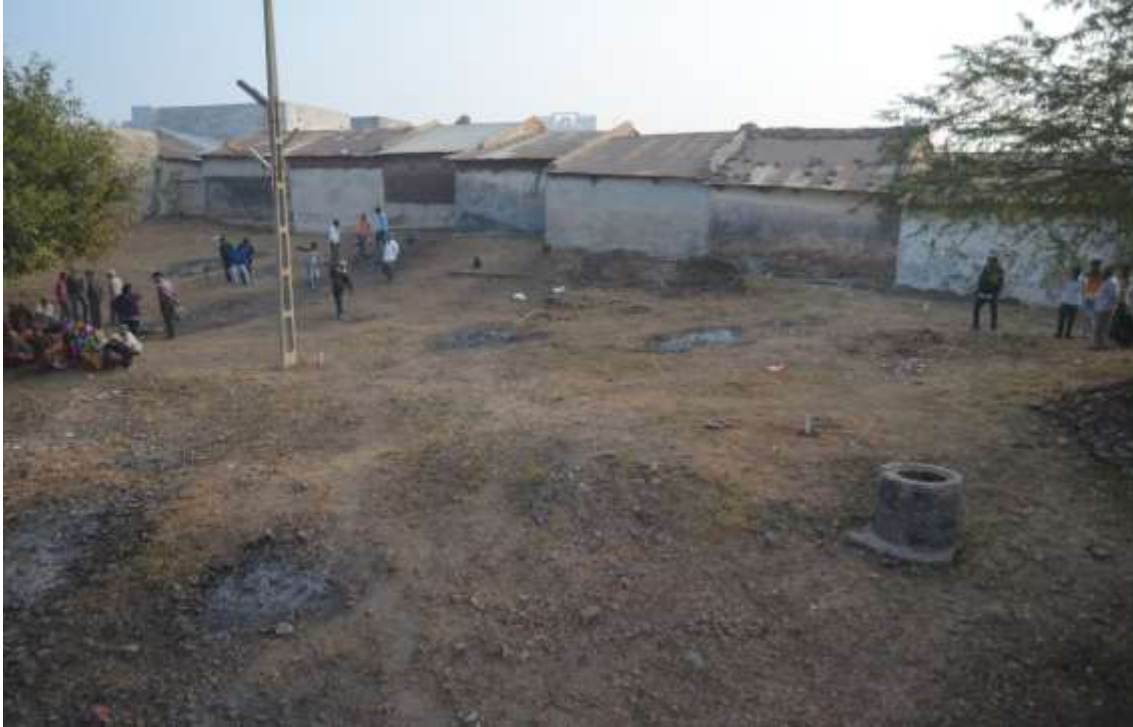
Figure 2: Preparation for laying out excavation trenches
