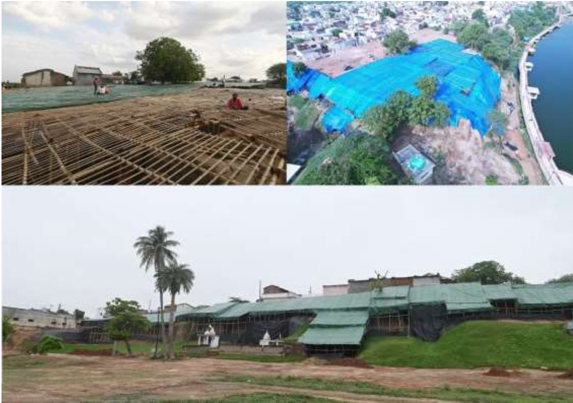
Figure 4: Temporary shed for the protection of excavated remains during monsoon
