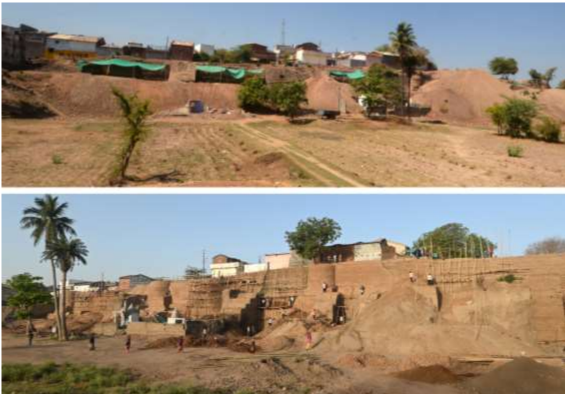
Figure 18: Long stretch of fortification wall - before and after
