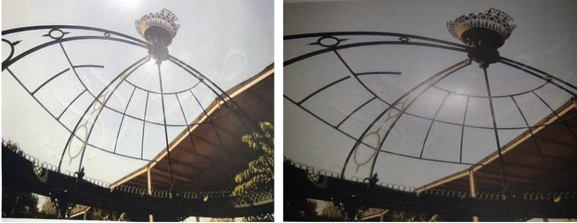
Figure 24: The remains of the dome's circumference with its metal beams of the music kiosk in Cairo's Azbakeyah Garden
