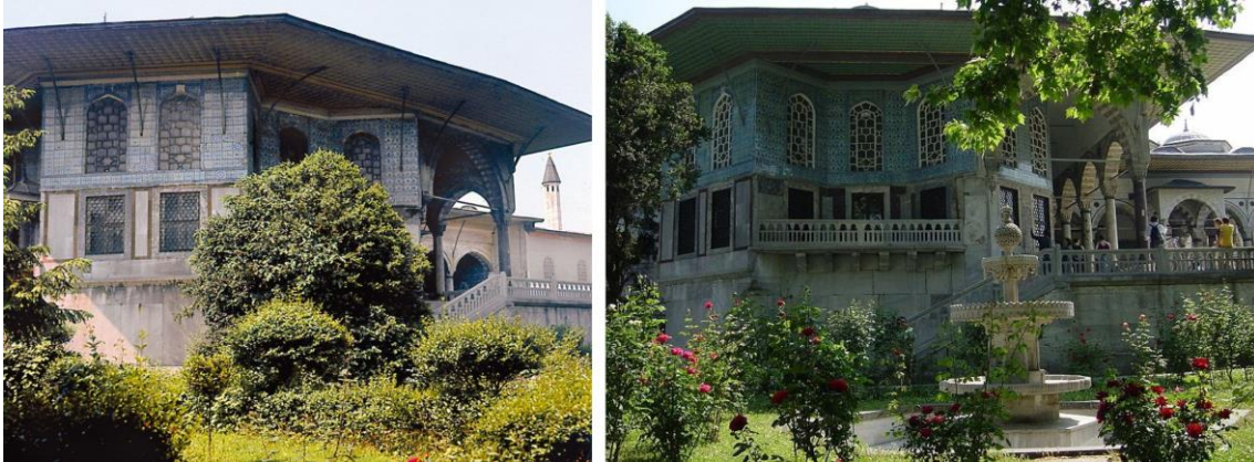
Figure 5: The pavilion of Revan in the fourth courtyard and the Topkapi Palace, Istanbul, Turkey (Courtesy: Hasan 2008)
